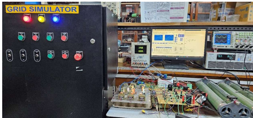
Fig. 5.11. Complete experimental setup for PV to Grid tied MOHC.
