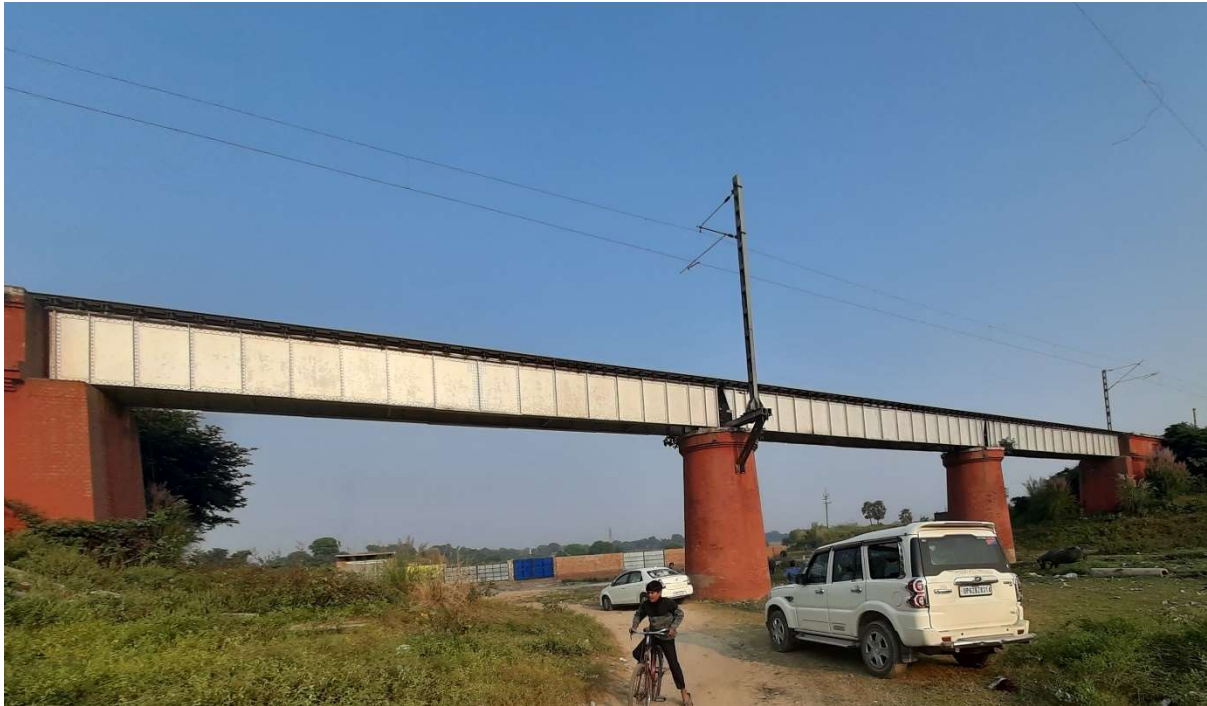
Figure 6.7: Case study 2: Steel Girder Bridge
