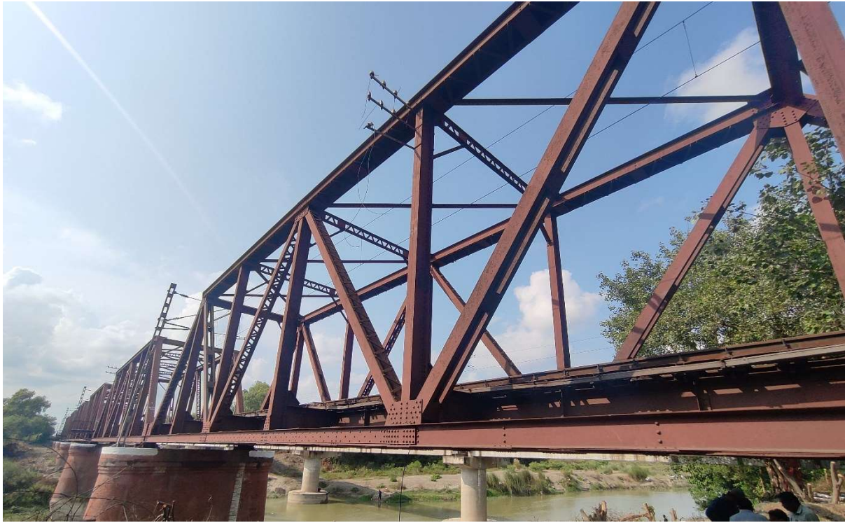
Figure 6.8: Case study 3: Steel Truss Bridge
