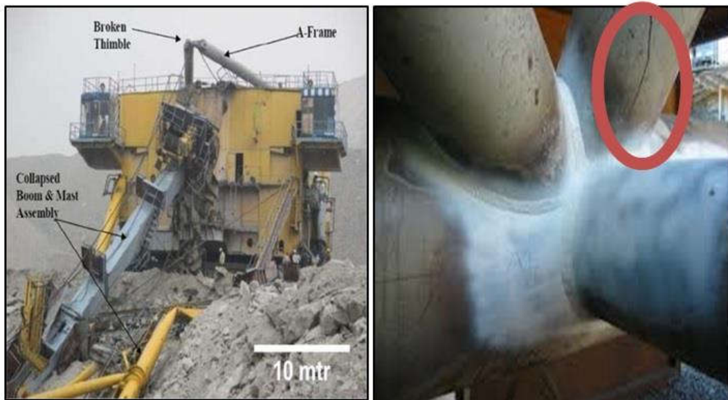
Figure 4.27 (a) Boom failures in an Indian coal mine and, (b) location of crack within the boom cluster
