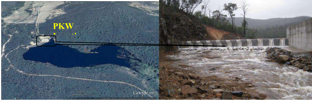
Figure 2. 6 Spatial Location of Loombah Dam (Australia) PKW (Ref: Google Earth)
