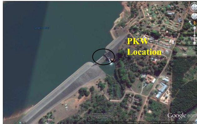
Figure 2. 5 Spatial Location of Tzaneen Dam PKW (Ref: Google Earth)
