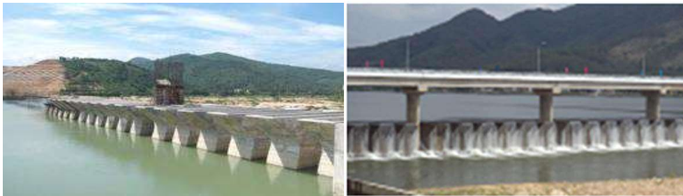
Figure 2. 7 Under construction and constructed PKW at Van Phong Dam (Vietnam)
