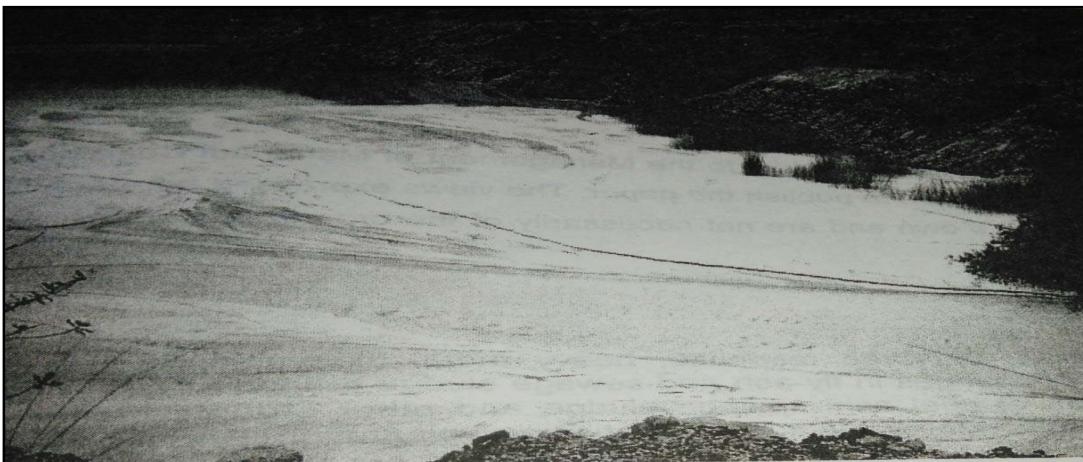
Fig. 2.3: Flyash mound formed in the used quarry of Balanda, OCM after disposal of ash slurry from TTPS
