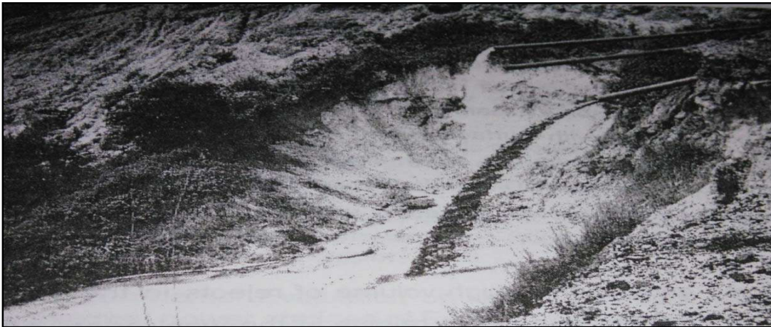
Fig. 2.2: Disposal of Flyash slurry through pipe line from TTPS into residual quarry of Balanda OCM, MCL
