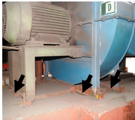
Fig: 3.42 Additional Stiffeners Welded on Base Frame
