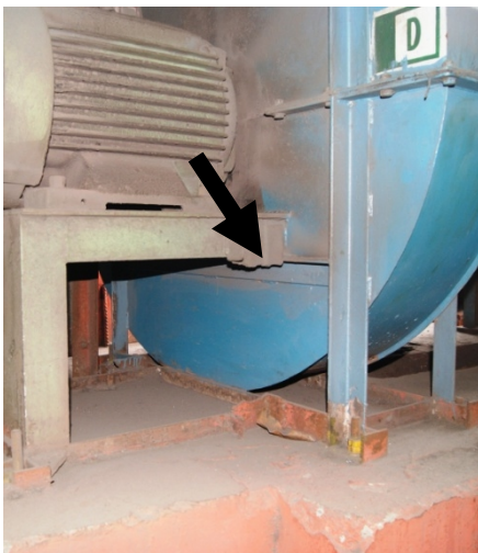
Fig: 3.41 Stiffeners Welded on Base Frame
