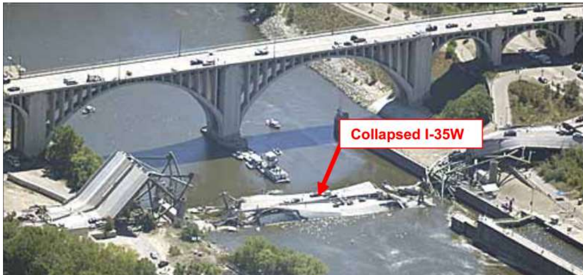
Figure 1.8: View of the collapsed I-35W bridge (A. Astaneh-Asl 2008)
