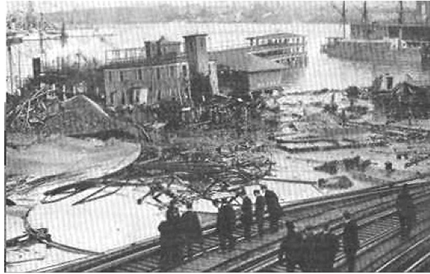
FIGURE 1.2: The Great Boston Molasses Disaster. Twenty-one people were killed, and more than 150 buildings were destroyed as the result of 2.3 million gallons of molasses flooding North Boston. Investigations indicated the probable cause to be brittle fractures.
