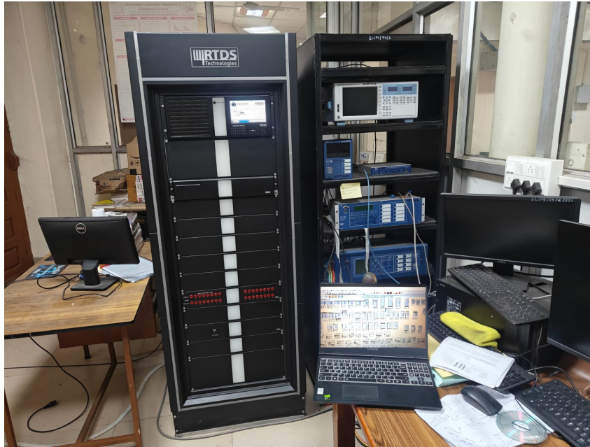
Figure II.2: IMAGE SHOWING RTDS CONNECTED TO WORK STATION
