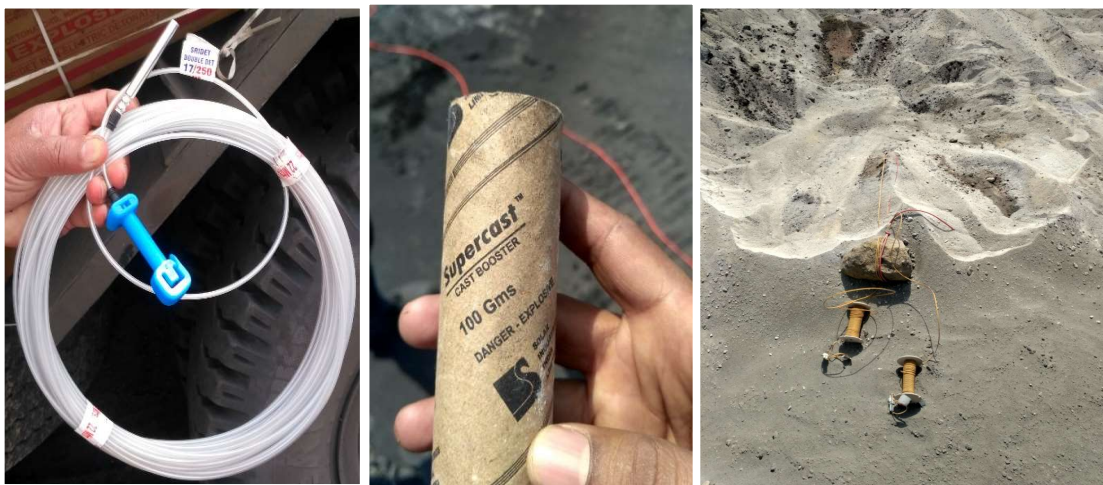
Figure 2.14 Applied delay, booster, and blast holes ready for blasting
