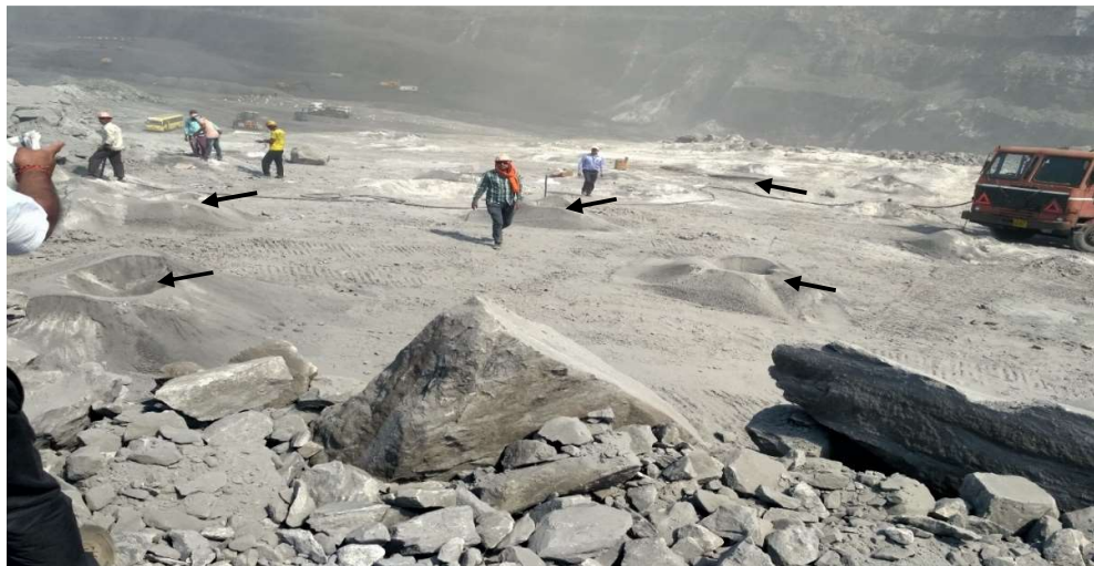
Figure 2.13 Preparation of blast holes in a patch
