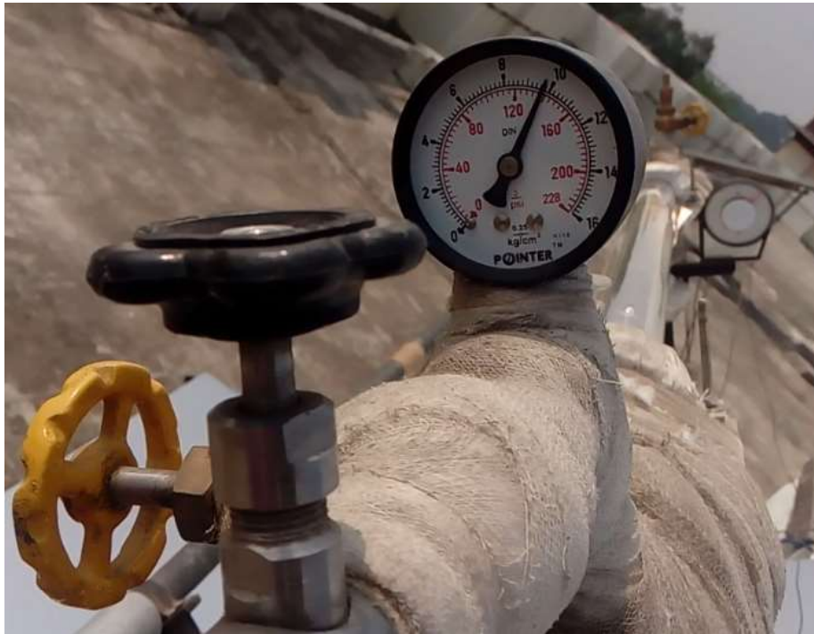
Figure 3.13: Photograph of steam pressure gauge to measure steam pressure inside the helical coil
