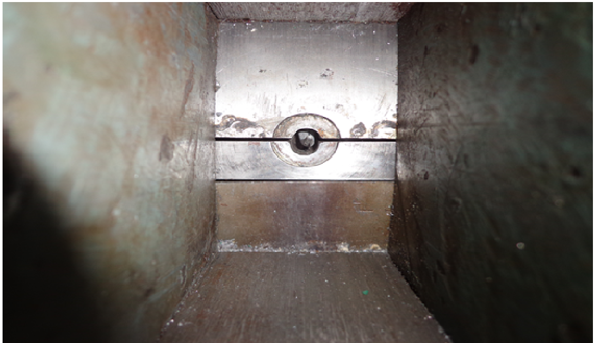
Figure 4.16: Material coming out of the abutment hole
