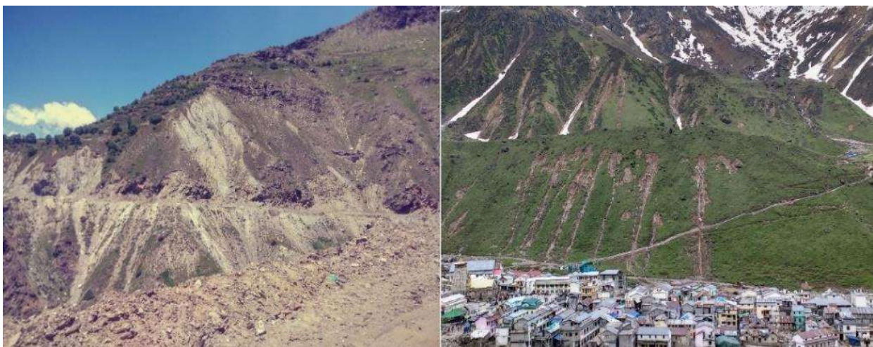
Fig. 4.3. Several localised debris flows observed during site investigations
