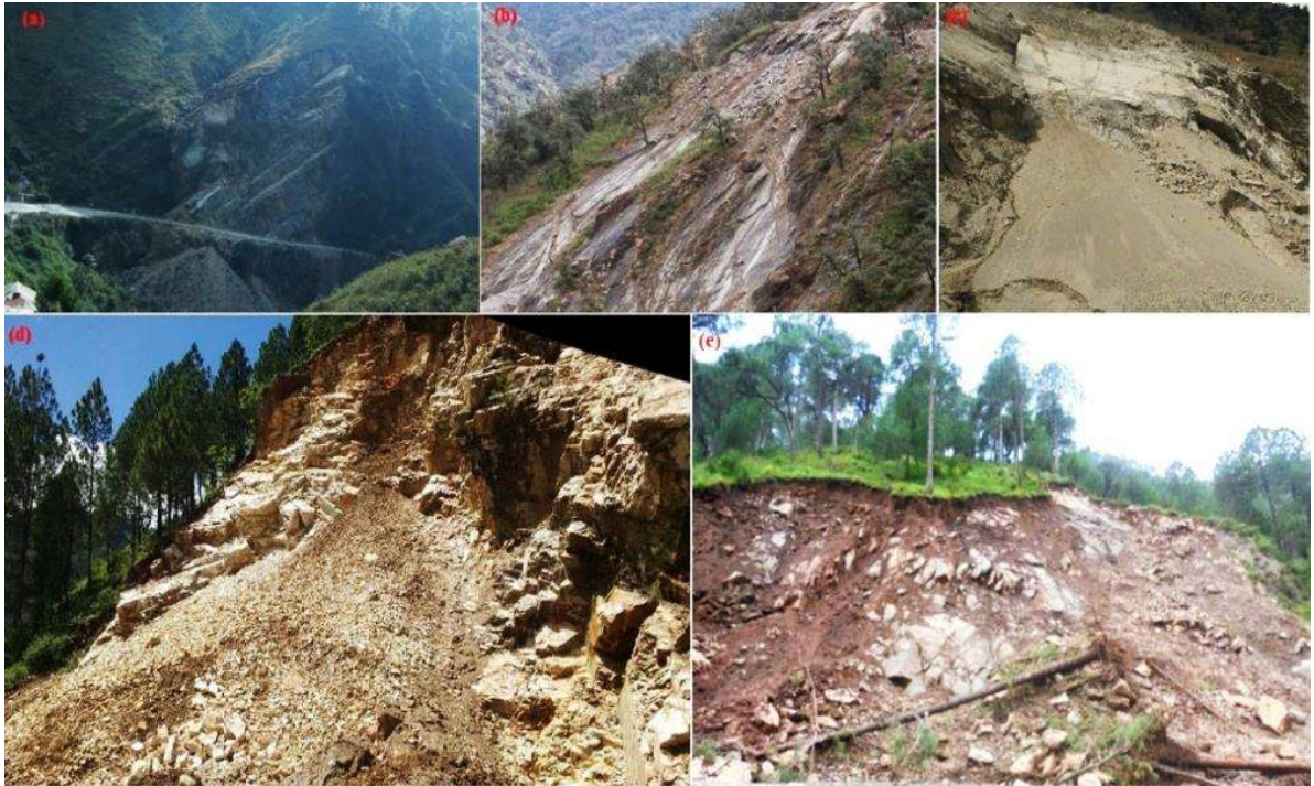
Fig. 4.5. Failure of residual soil mass overlying a bedrock as observed in several locations in the study area
