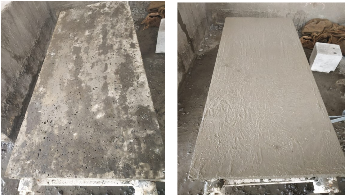
Figure 3.20 Deck slab before and after plastering.
