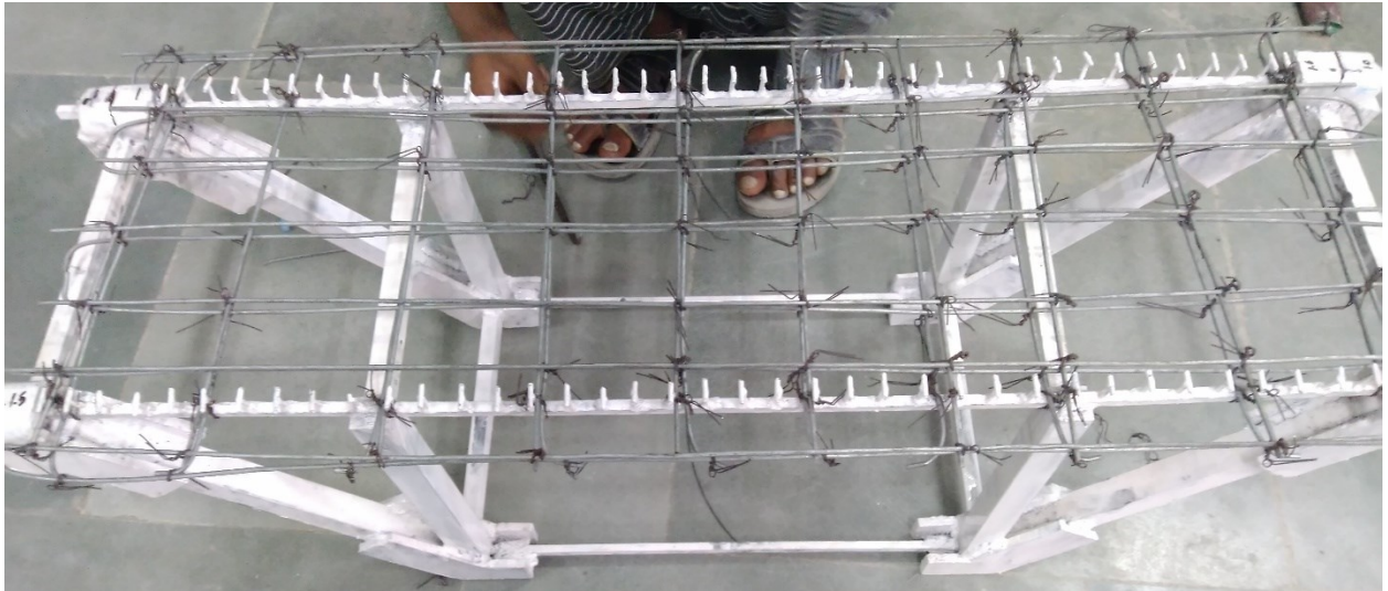
Figure 3.18: Shear studs and deck reinforcement.
