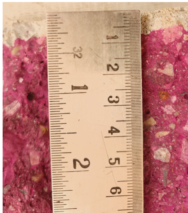
Figure 6.38: Carbonation depth of F60RC
