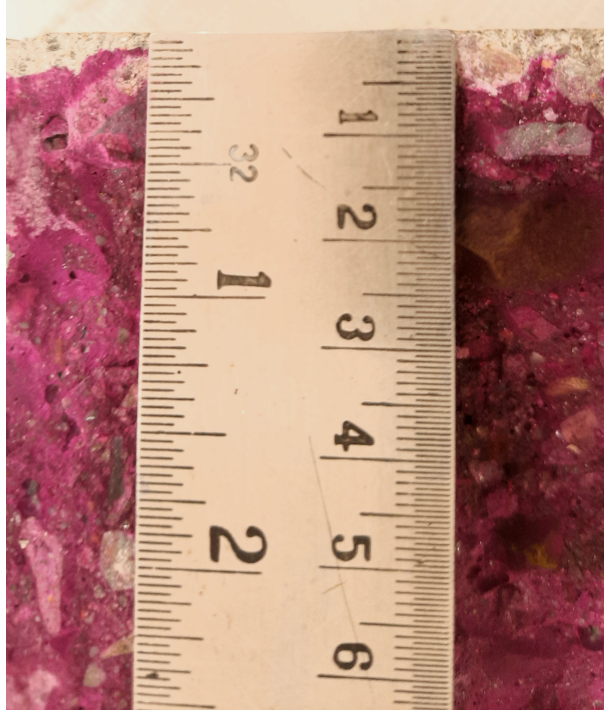
Figure 6.42: Carbonation depth of C100F30RC
