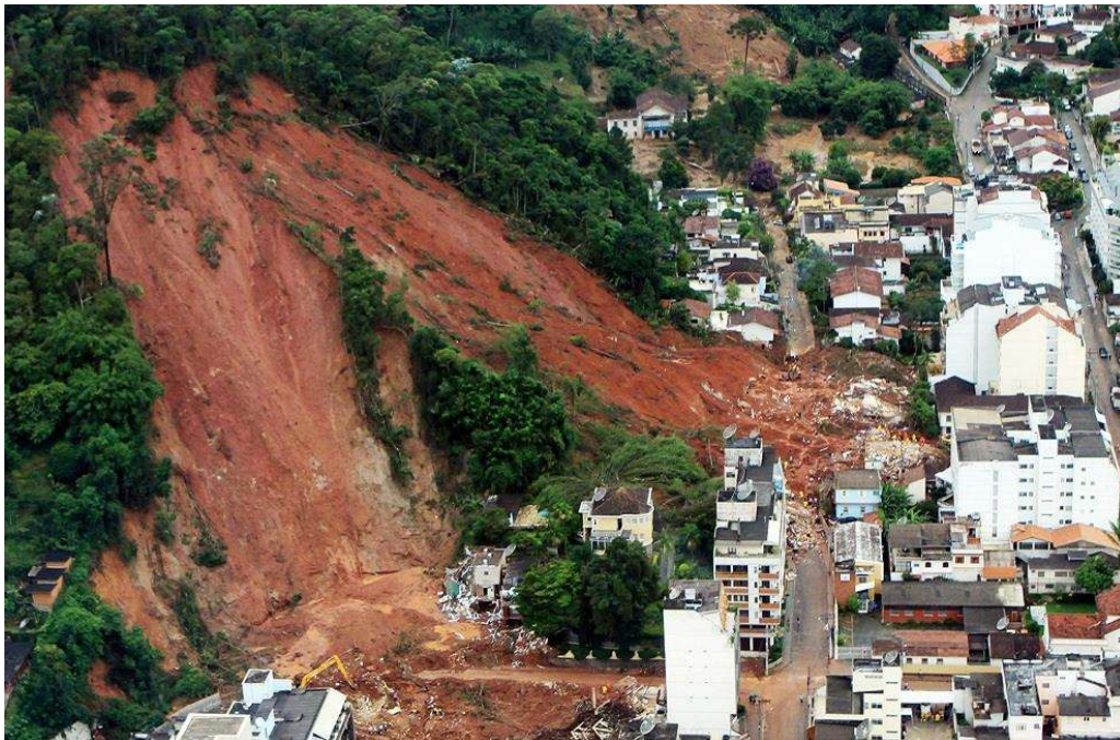
Fig. 2.9. A severe debris flow affecting downslope settlements (Haugen and Kaynia 2008)
