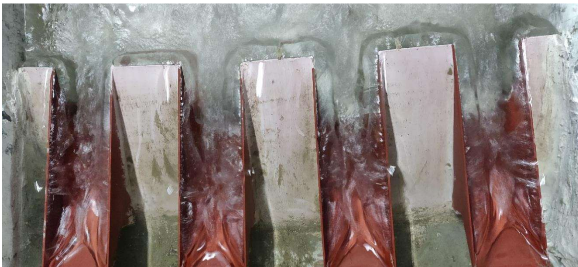
(a) Continuous water film running around inlet-outlet of RPKW
