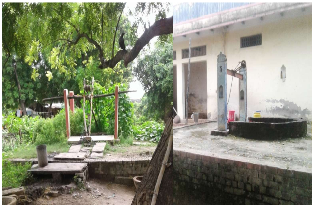
Figure 4.11 open dug well for groundwater sampling
