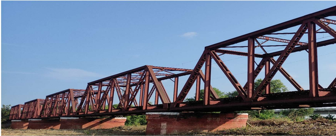
Figure 3.12: Steel railway bridge in the Bareilly-Rampur section
