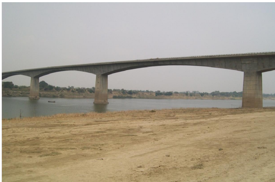
Figure 5.6: Photograph of Viswasundari Bridge with bridge piers
