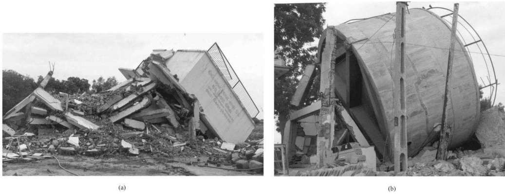
Fig. 2.3: Collapsed water tank stagings in Manfera village. (b) Damaged water tank staging in Bhachau. [Rai, 2003]
