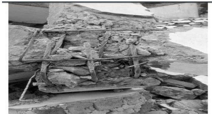
Fig. 2.3: Collapsed water tank stagings in Manfera village. (b) Damaged water tank staging in Bhachau. [Rai, 2003]
