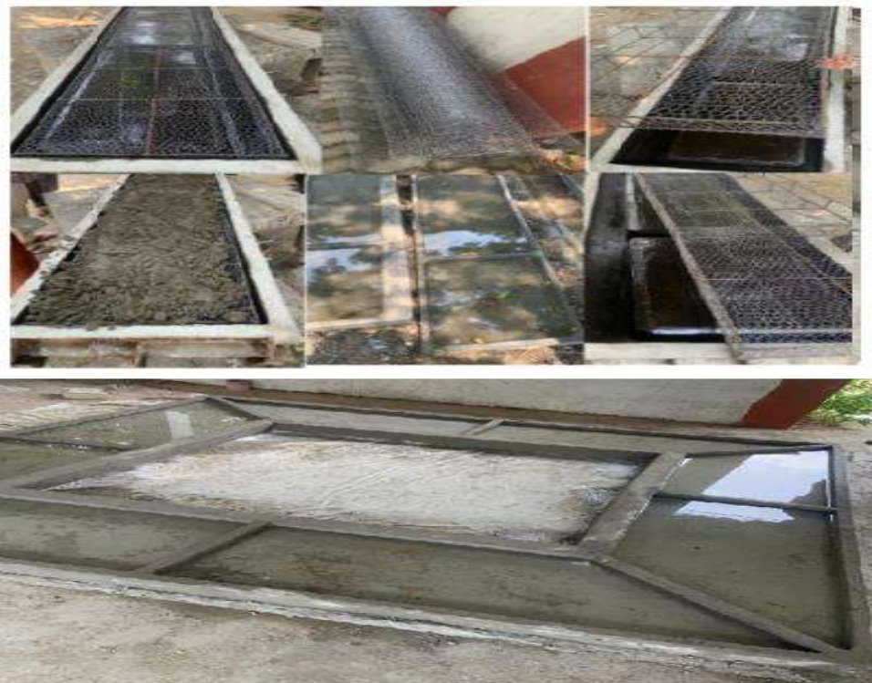
Fig. 1.15: Pictures of Casting of ferrocement at T.M.M Building Centre and ferrocement Factory Tilothu Rohtas Bihar India
