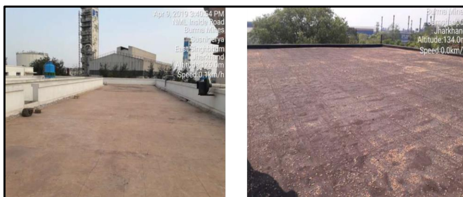
Figure 6.5- (a) and (b): proposed installation site roof photographs.
