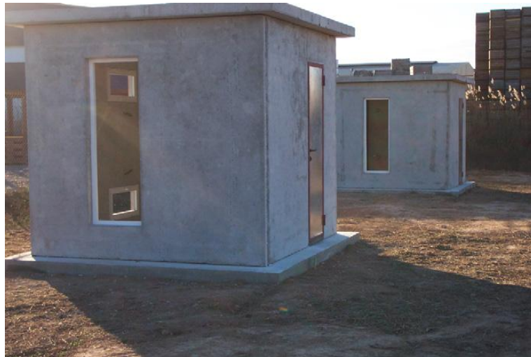
Figure 2.5 Developed cubicles using MPCM for analysis (79)
