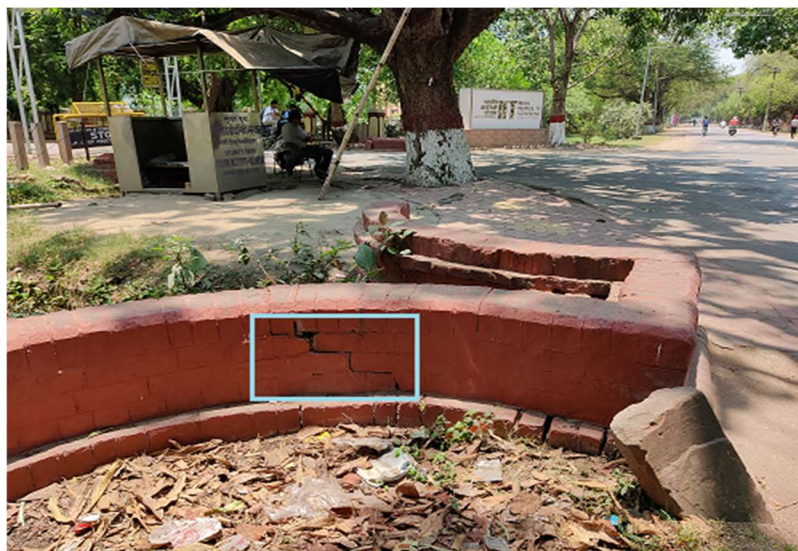
Figure 5.16: Existing old masonry culvert bridge at Banaras Hindu University, India
