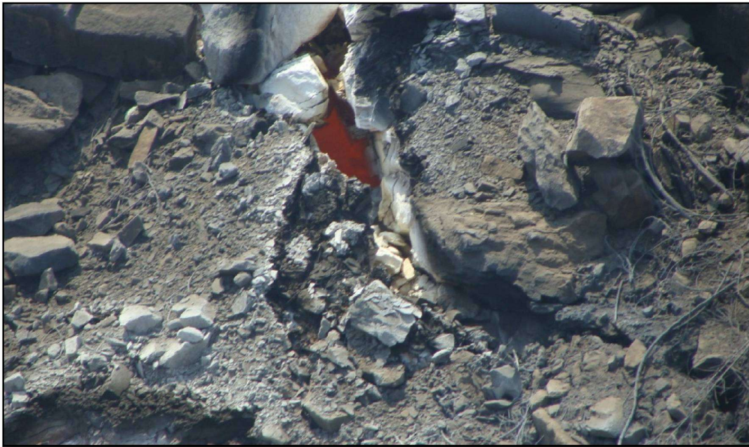
Fig: 14 Visible CSF at the fissures depicting the development of fire chamber The CSF is visible in the weak zones at the fissures & cracks.
