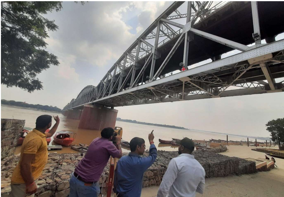
Figure 4.10: Deflection measurement with a digital total station (TS) at the bridge site
