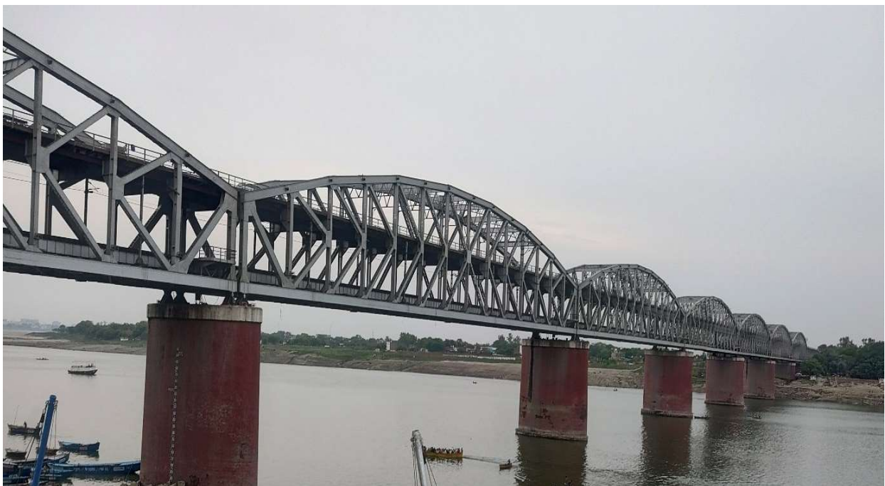
Figure 4.1(a): Steel railway bridge in the Pt. DD Upadhyaya -Varanasi section
