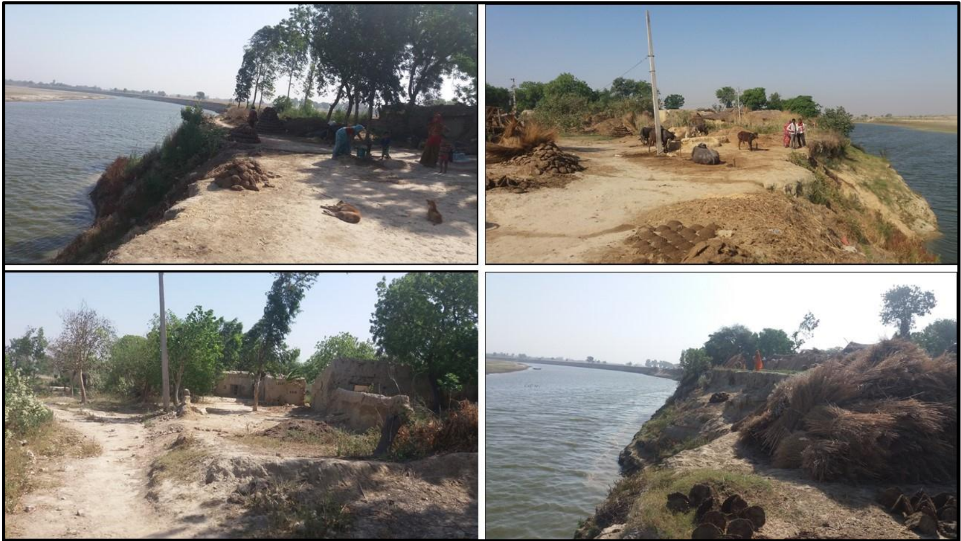
Figure 7.8 Severe bank erosion with fracturing and collapse of the bank
