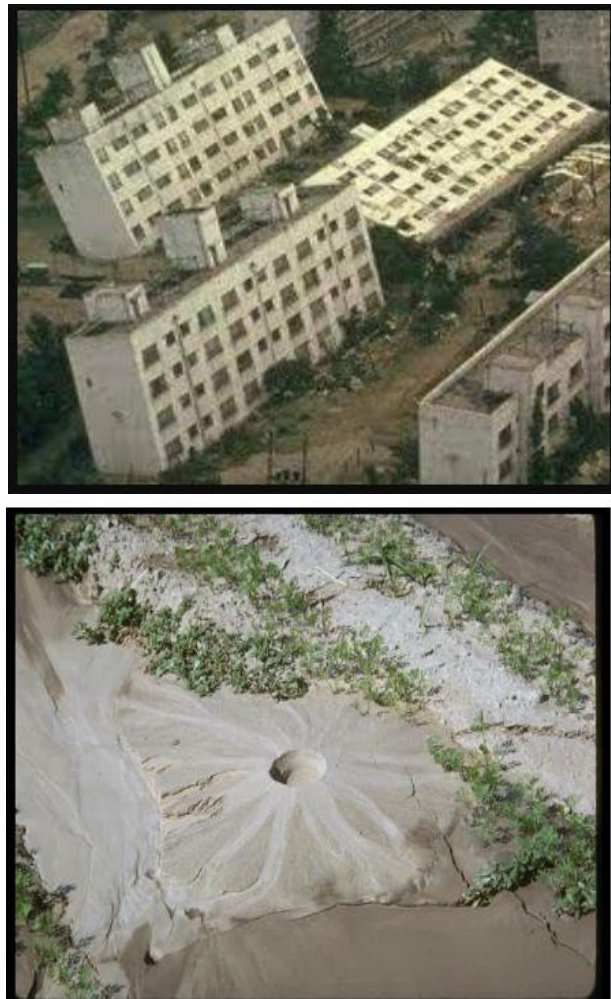
Fig. 1.1 (a) Toppling of a building during Niigata earthquake in 1964 (b) Sand boil during California, earthquake, 1979 (Steinbrugge Collection, Earthquake Engineering Research Center, University of California, Berkeley)
