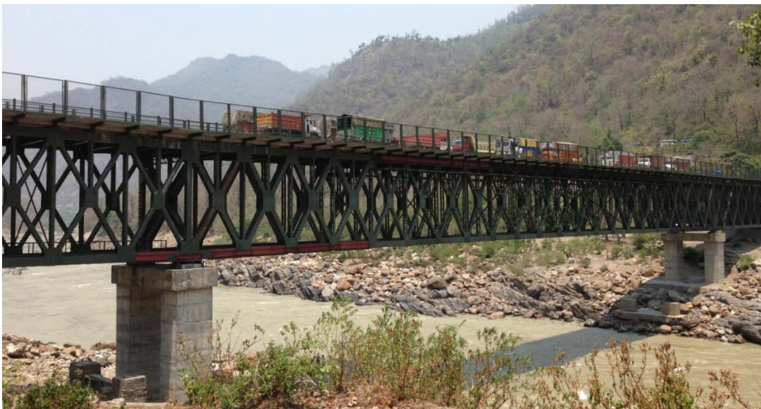
Figure 3.17 Garudchatti bridge over Alaknanda river, India
