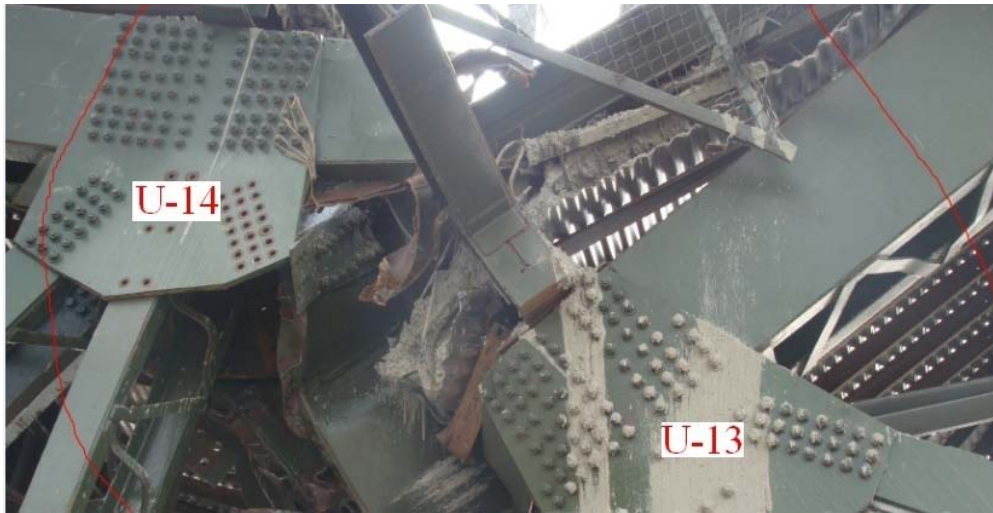
Figure 3.19 Intact gusset plates at joints U13 and U14
