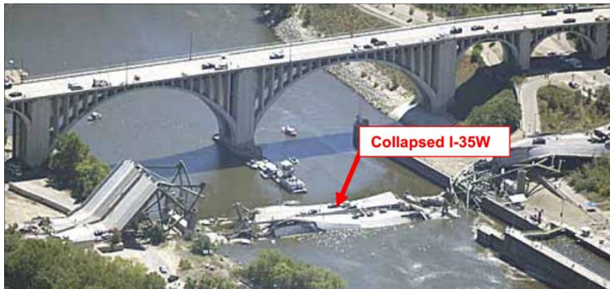
Figure 3.1 View of the collapsed I-35W bridge (A. Astaneh-Asl, 2008)
